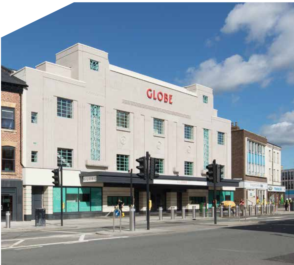
The restored elevation of the Globe complete with the 1935 neon sign
